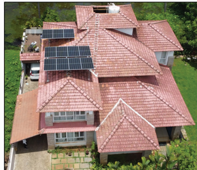
Residential Solar Power plant
